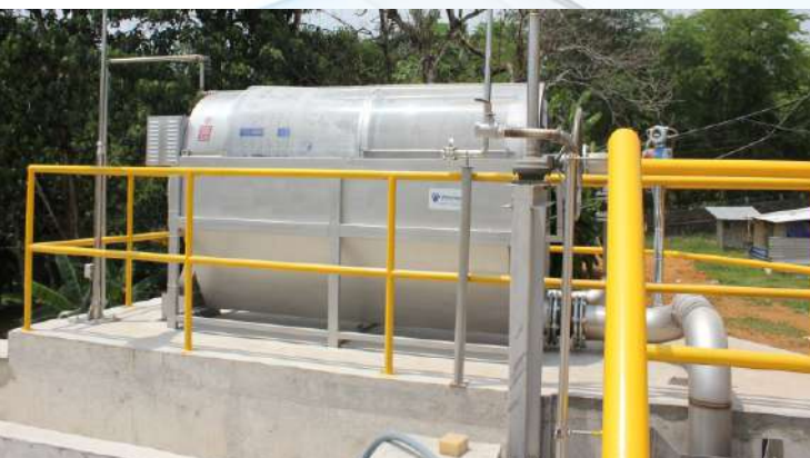
Drum Screen installation for waste water recovery plant in Sri Lanka for flow 1000 mcd
