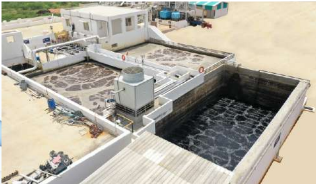
BIO MBR and Reverse Osmosis for 1400 mcd in India BIO MBR y Ósmosis Inversa para 1400 mcd en India
